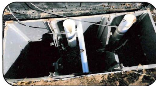
* Overhead view of 3-chamber box actively charging—note water flowing over first stop log (right) from the field and no water flowing over the second stop log (left) indicating an active charge event
