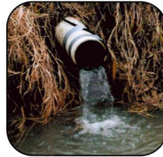
* View of the free flowing drainage comparison site
